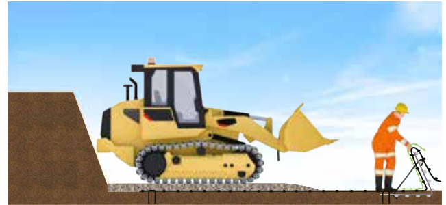
Forming the face of the reinforced wall
