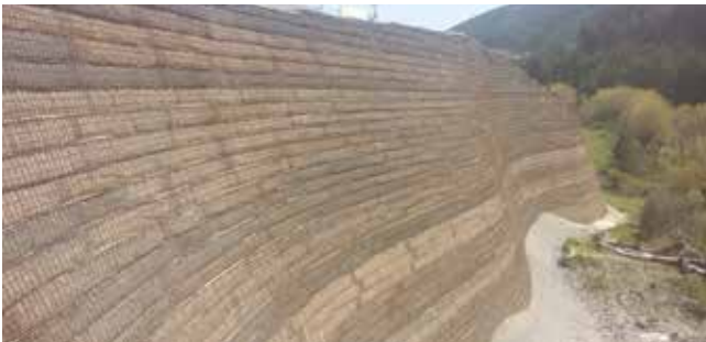
Gaining space at narrow expropriation areas
