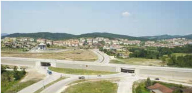
Bridge approach walls
