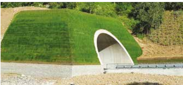
Landscaping of tunnel portals
