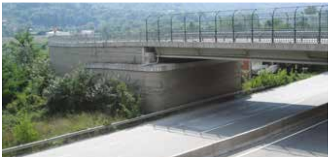
Bridge abutment walls
