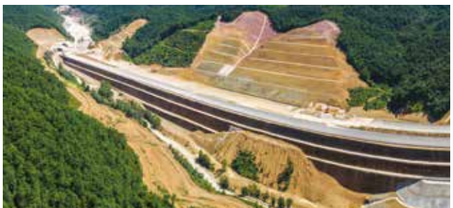
Long and high MSE walls
